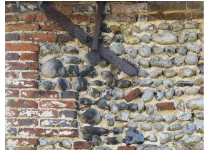
Regular overspilling of water from missing, damaged or inadequately sized rainwater goods causes damage to the historic fabric
