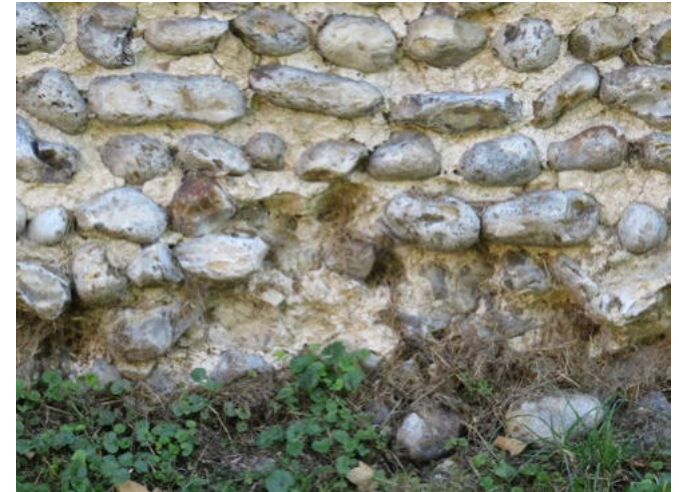
Eroded pointing causes loss of flints
