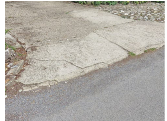
Large concrete splay
